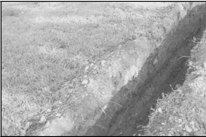
Plate 1. Trench showing buried surface beneath Terrace fill.
