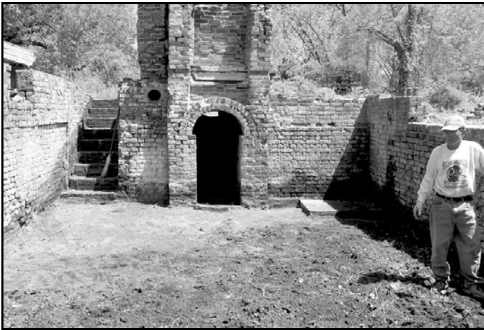
Mt. Air basement after cleanup!
