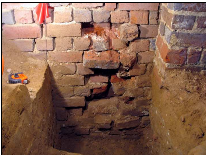
Me? I dug under the floor boards! But, I found this old foundation keyed into the main cellar wall!
