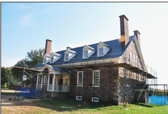
Gunston Hall (Renovation in Progress)
