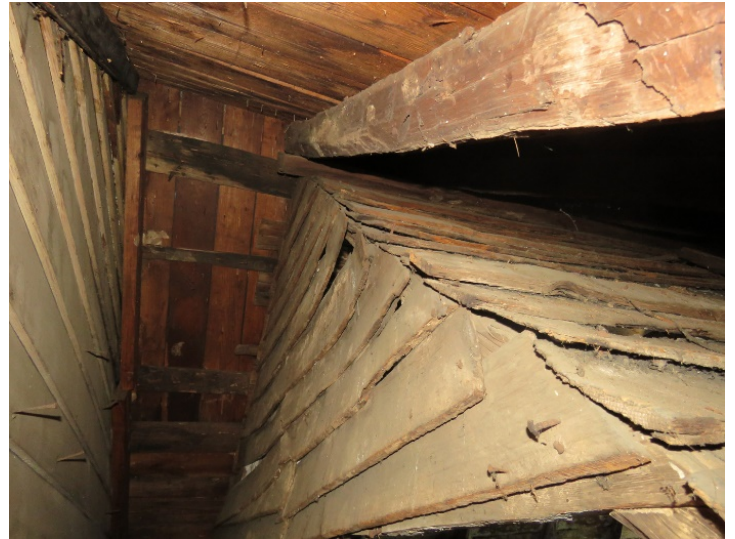
Second story gap between the original log house on the right and the 1880s addition on the left
