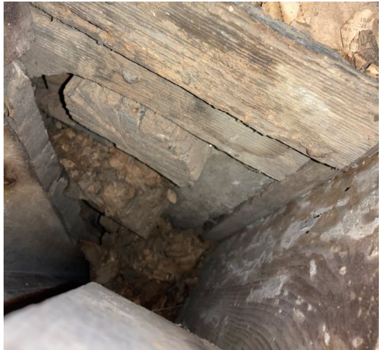
Hewn and notched beams under the 1880s house. Shaft revealing structural details on 1740s log house.
