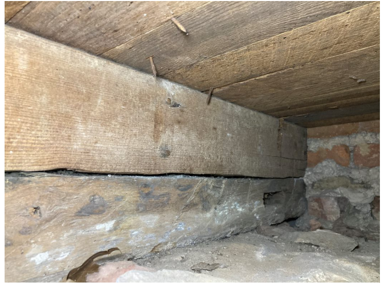
Hewn and notched beams under the 1880s house. Shaft revealing structural details on 1740s log house.
